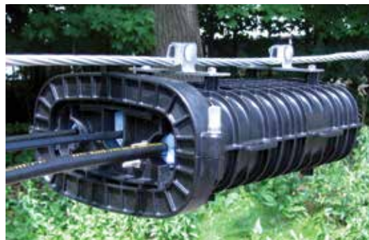
Low Clearance Strand Mounting Bracket
